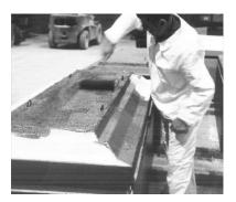
Water Based Damp Proof Coating for Concrete
